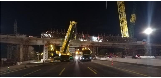
Figure 14. Deconstruction general view.
