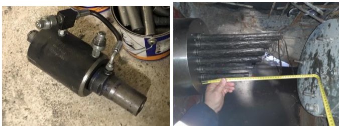
Figure 20. On the left hand, mono strand jack of reduced dimensions. On the right hand, free space between anchors block. Detail while the stressing operation.
