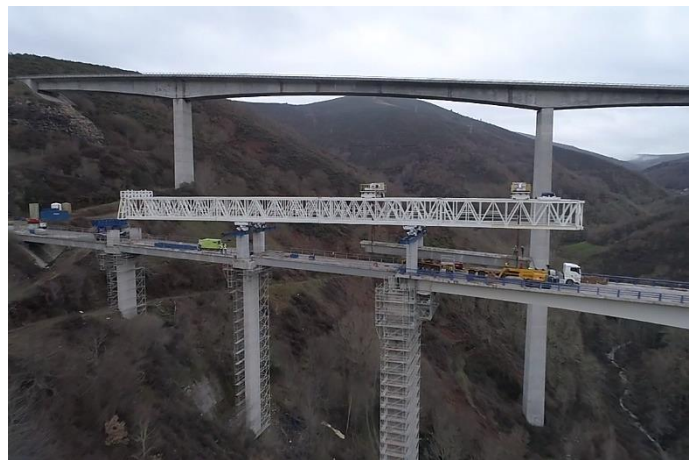
Figure 9. Ruitelán first deconstruction V-shape beam with a launching girder.
