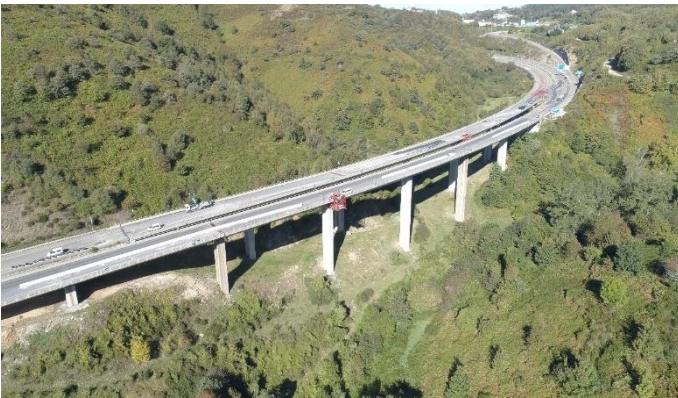
Figure 15. Castro viaducts general overview.
