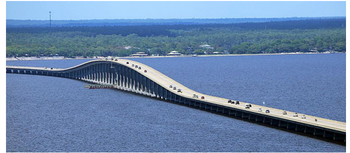
Figure 4. Mid-Bay Bridge general overview. Source: https://www.mid-bay.com/about-us-2/mid-bay-bridge/
