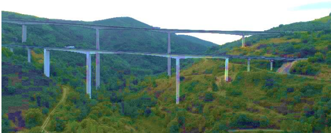
Figure 6. Ruitelán (down) general overview. At the left, north approach viaduct.
