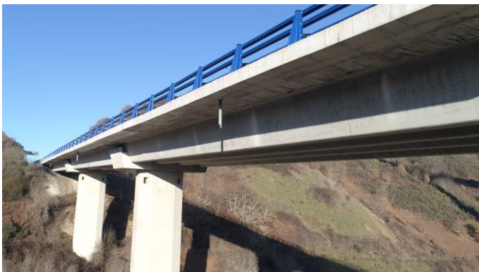
Figure 7. Ruitelán detailed view of north access viaduct.
