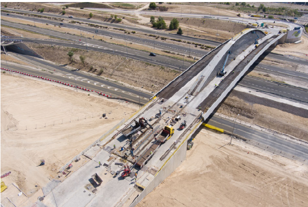
Figure 21. Slab concrete in 12 m central section
