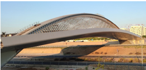
Figure 5. Structure overview during construction
