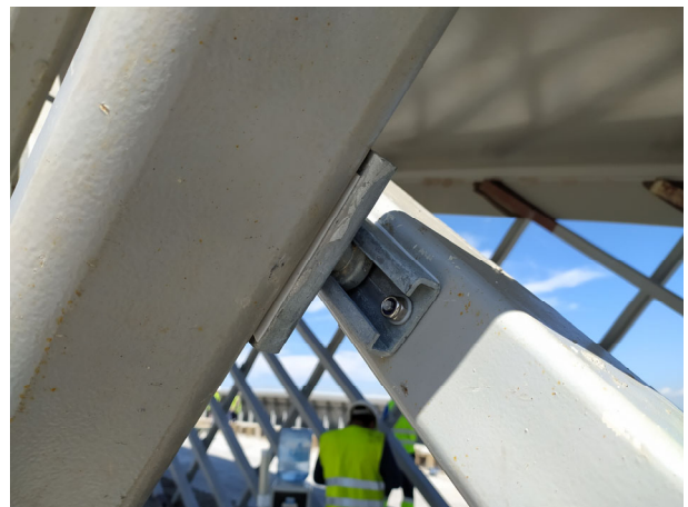
Figure 12. Wind-induced vibrations control element
