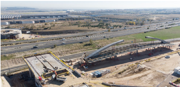
Figure 18. Steel structure assembled in work
