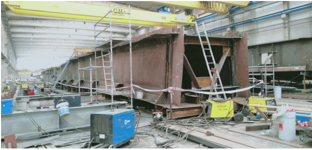
Figure 17. Steel structure manufactured in workshop
