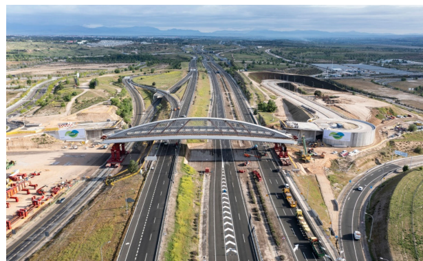
Figure 20. Rotation and transported of bridge's central segment
