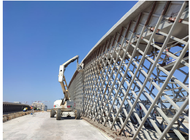
Figure 11. Diagrid assembly
