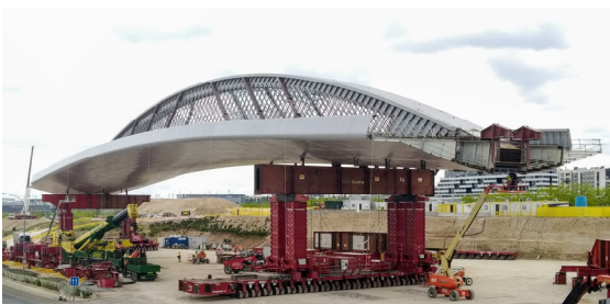
Figure 19. Central segment of the bridge transported with SPMT
