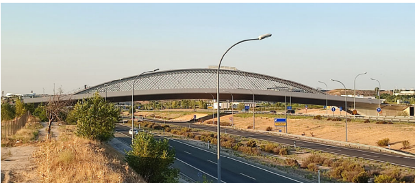
Figure 22. Bridge construction overview
