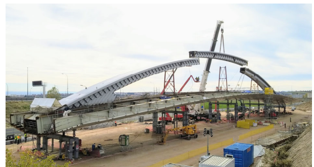
Figure 9. Lifting of arch central section
