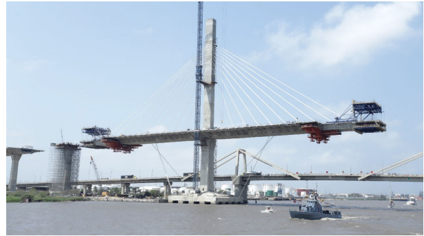
Figure 15. Cable-stayed section of the New Pumarejo Bridge during execution
