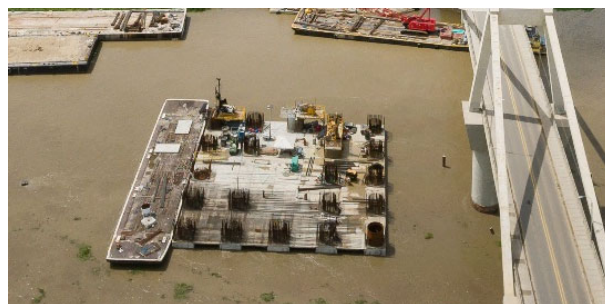
Figure 13. P14 pile cap during its execution
