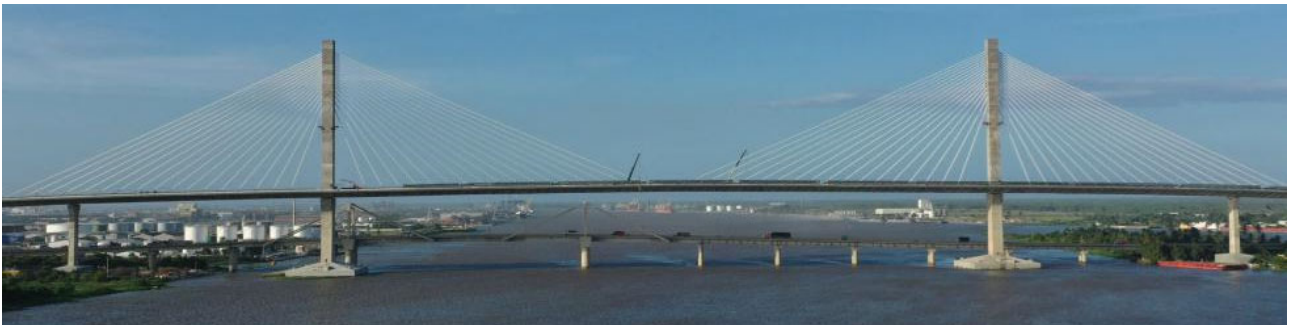
Figure 6. Side view of the cable-stayed section of the New Pumarejo Bridge built
