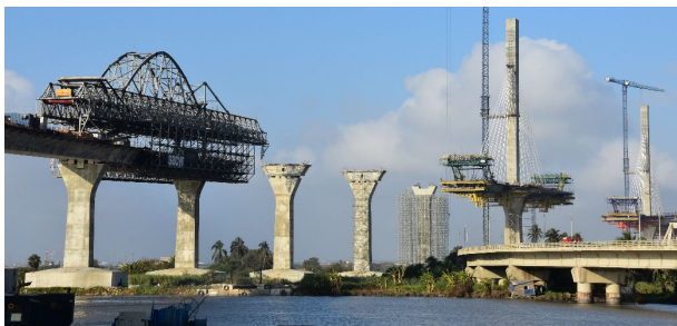
Figure 12. Piers of the right access viaduct during its execution
