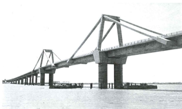
Figure 1. View of the Pumarejo Bridge from 1974
