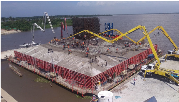
Figure 9. P14 pylon foundation during its execution
