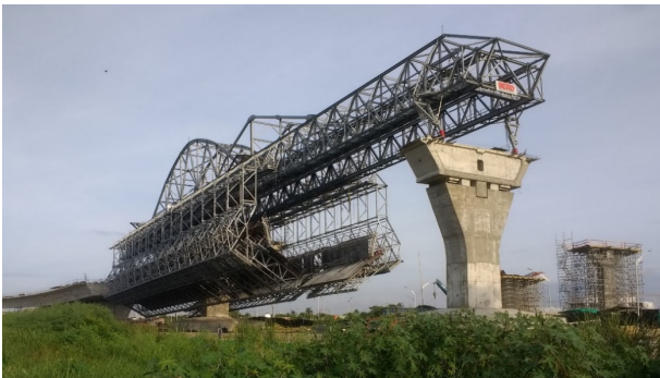
Figure 14. Execution process of the access viaducts with MSS
