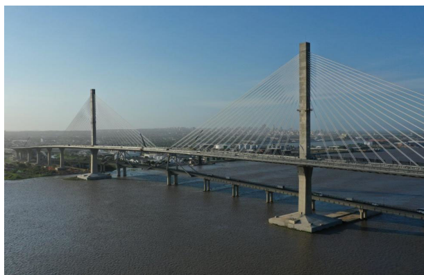
Figure 2. View of the New Pumarejo Bridge
