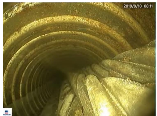
Figure 12. Photograph of the interior of the duct showing the incomplete filling by the grouting.
