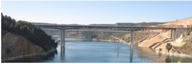
Figure 32. Contreras viaduct, 170-meter span composite truss.
