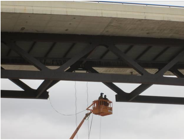
Figure 36. Replacement of the damaged element.
