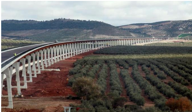
Figure 27. Archidona viaduct (Spanish HSRL). 3150 meters between expansion joints at abutments.
