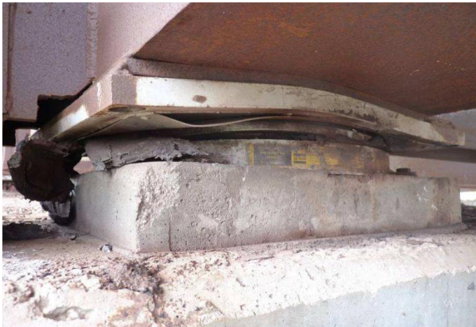
Figure 33. Contreras viaduct: bearing devices under out-of-service conditions.
