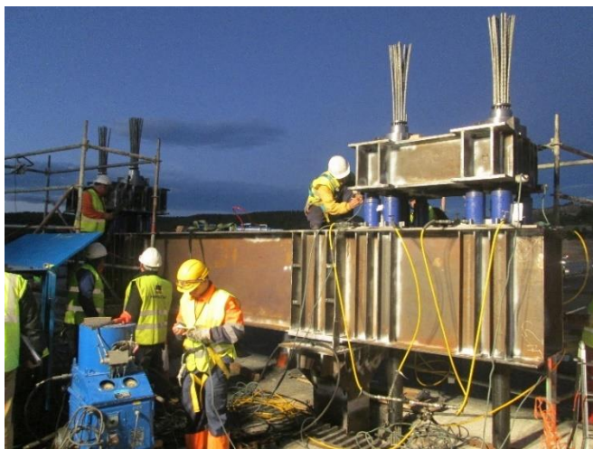
Figure 34. Contreras viaduct: cable lifting from the carriageway in order to facilitate the bearing replacement, as it had not been planned from pier caps (2014).
