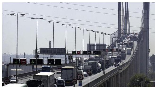
Figure 48. Traffic-jammed Centenary bridge (100000 vehicles/day).
