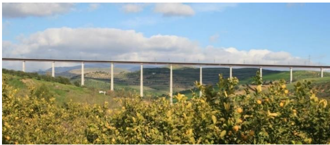
Figure 28. Arroyo de las Piedras viaduct (Spanish HSRL). 1210 meters between expansion joints at abutments and piers of up to 95 meters height.
