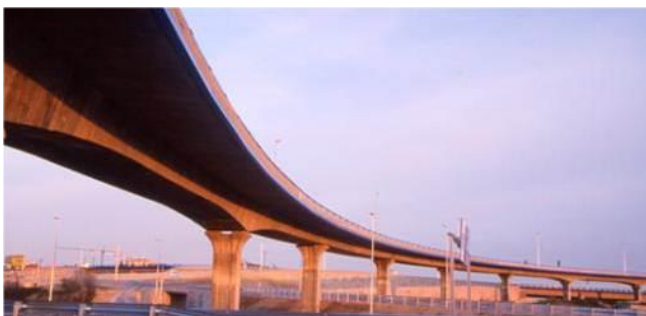
Figure 23. Precast, varying depth continuous viaduct at the M50 to M501 connection in Madrid.
