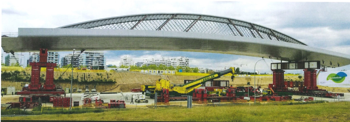
Transportation of the 128.65m-long central section of La Concordia Bridge took place in April
