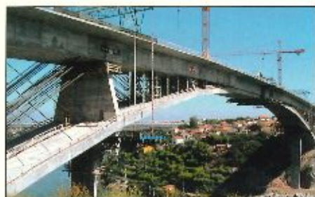
Fig. 4: View of the bridge before temporary elements were dismantled
