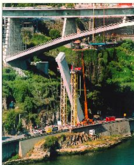
Fig. 5: Removal of the temporary pillar on the Porto side of the bridge
