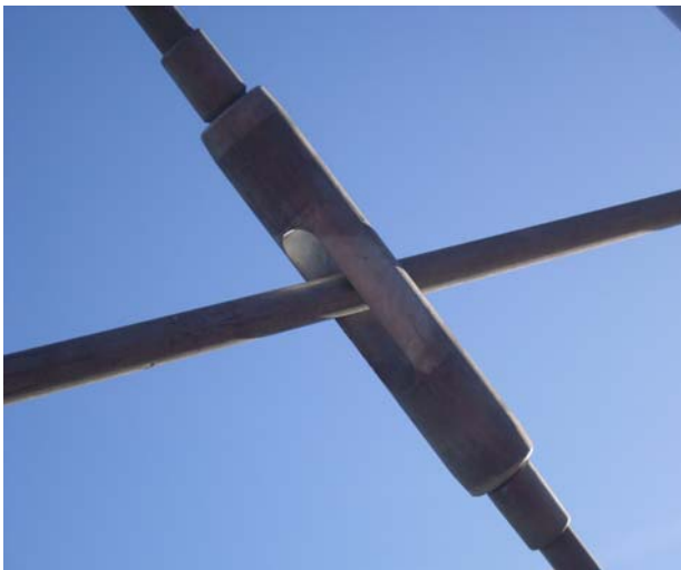
Fig. 12 N-II footbridge hanger crossing device.
