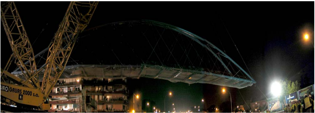
Fig. 13 Erection of N-II footbridge.
