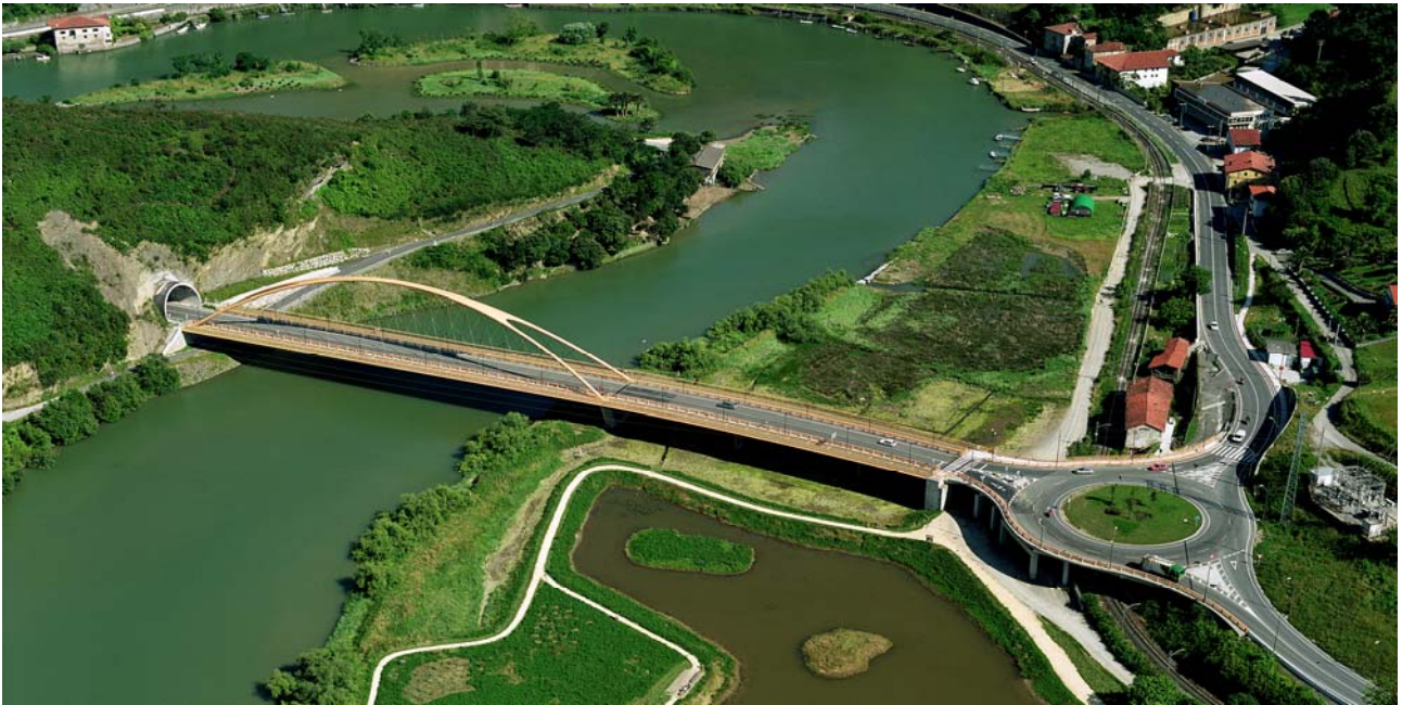
Fig. 14 Bird's eye view of the bridge and the access viaduct.
