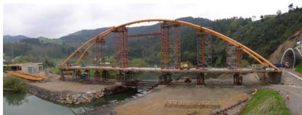
Fig. 29 View of the arch and deck while shored.
