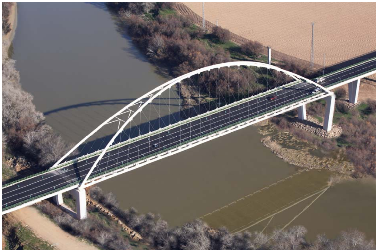
Fig. 32 Bird's eye view of the arch bridge over River Guadalquivir.
