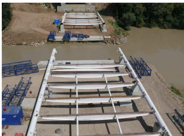
Fig. 38 Artificial embankments and steel deck assembly operations.
