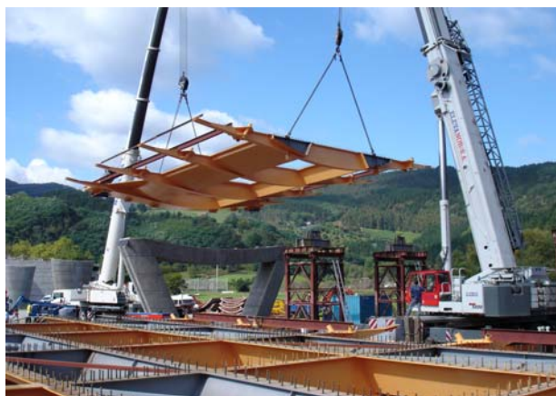
Fig. 28 Erection sequence of a steel deck segment.
