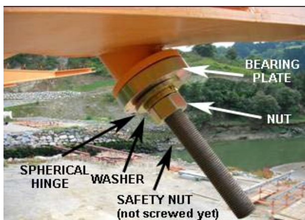
Fig. 27 Lower (hanger-deck rib) anchorage.
