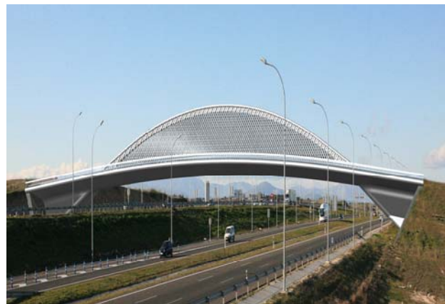
Fig. 45 Front view of the Valdebebas Bridge (render).
