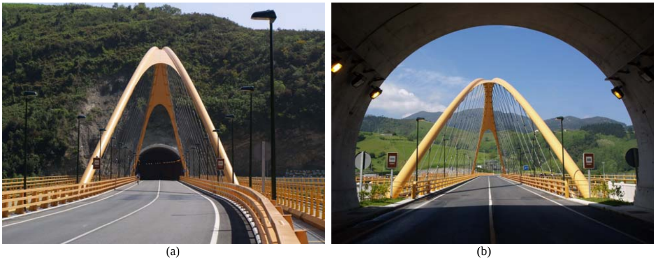
Fig. 15 Arch view from outside the tunnel and from within the tunnel.
