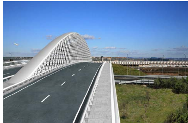
Fig. 44 Lateral view of the Valdebebas Bridge (render).
