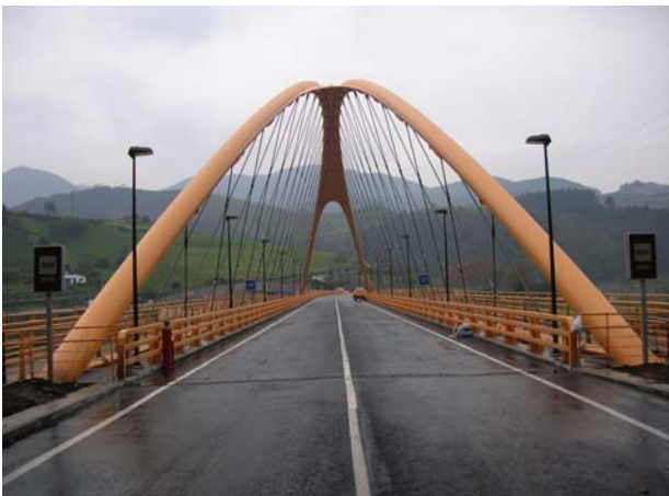
Fig. 23 View of the arch bridge from abutment 2 (tunnel).
