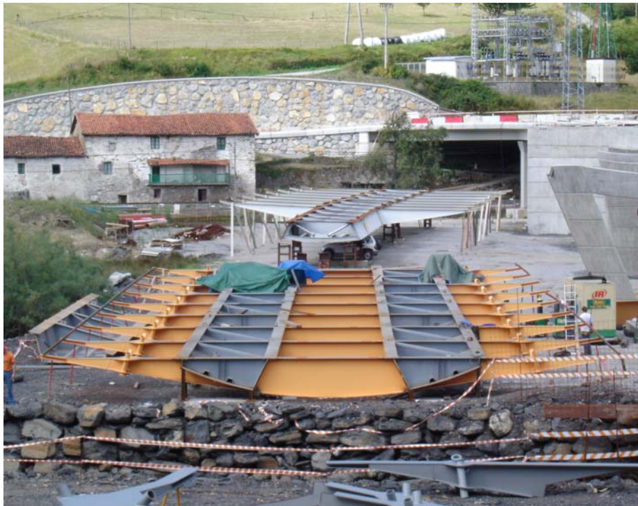
Fig. 21 View of the arch bridge's deck (foreground) and the access viaduct's deck (background) prior to their erection.
