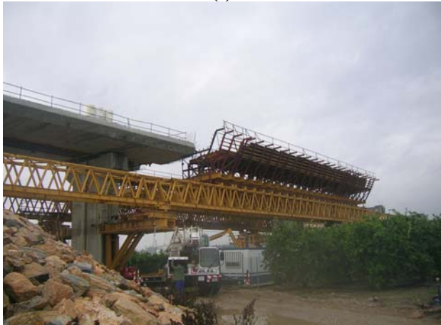
Fig. 31 Slab cross-section after widening and view of erection with falsework.
