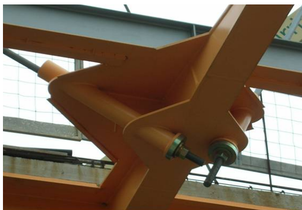
Fig. 26 Hanger lower anchorage close-up.
