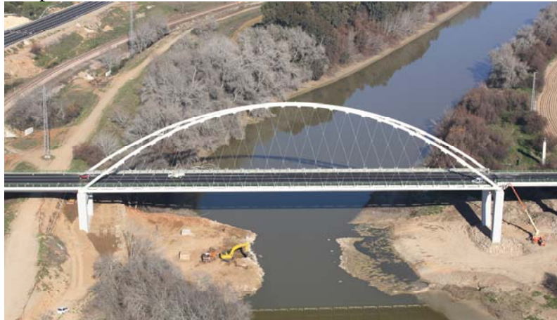
Fig. 6: Aerial View of “Palma del Río” Bridge over Guadalquivir River
