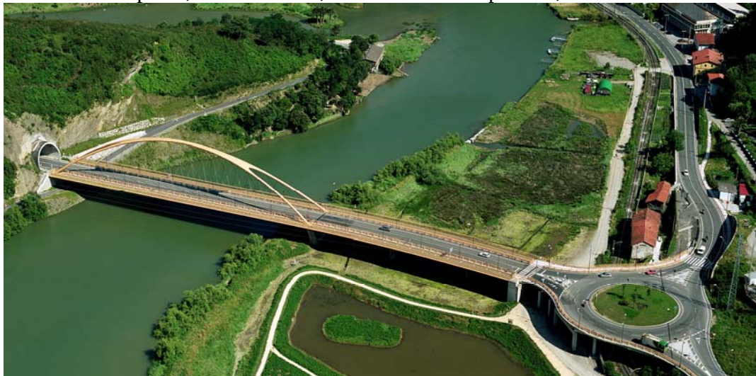
Fig. 5: Elevation view of the bridge over Deba River
