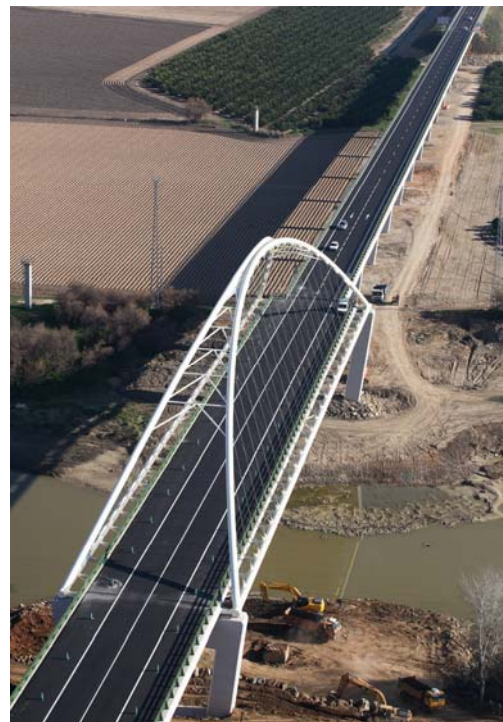
Fig. 8: Aerial view of the bridge
