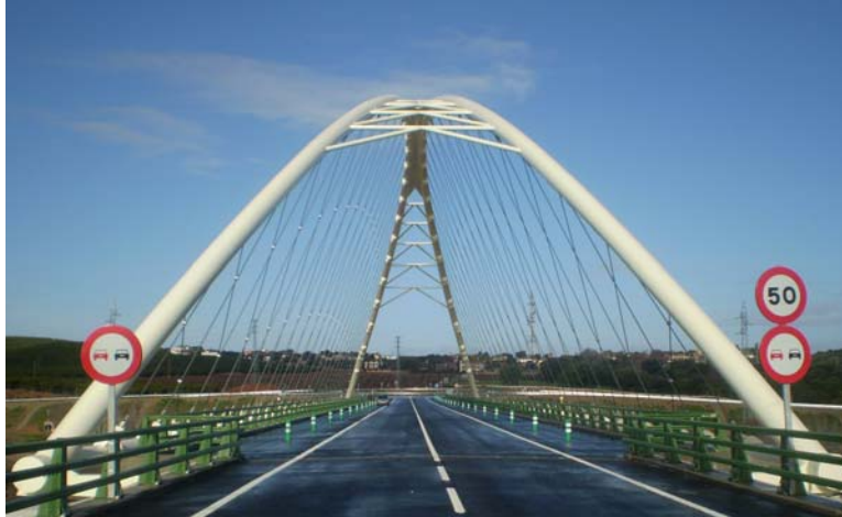
Fig. 9: Frontal view of the arches and the upper bracing.
