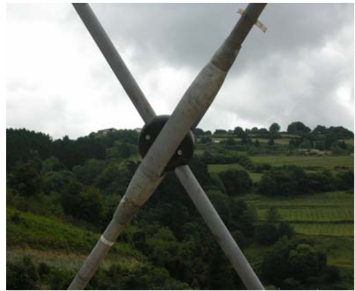
Fig. 13: Deba's rod hanger crossing device
