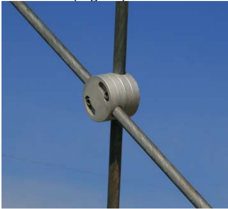
Fig. 12: Palma del Río's cable hanger crossing device
