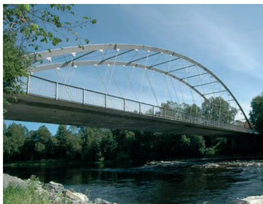
Figura 1. Puente de Steinkjer(1963) Figure 1. Steinkjer Bridge (1963)
