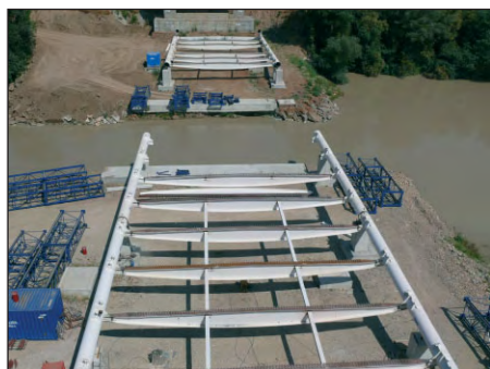
Fig. 12: View of the embankments of both sides of the river and the first segments of the steel framing for the deck
