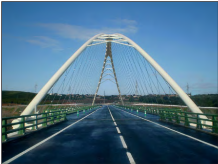
Fig. 8: Frontal view of the arches and the upper bracing
