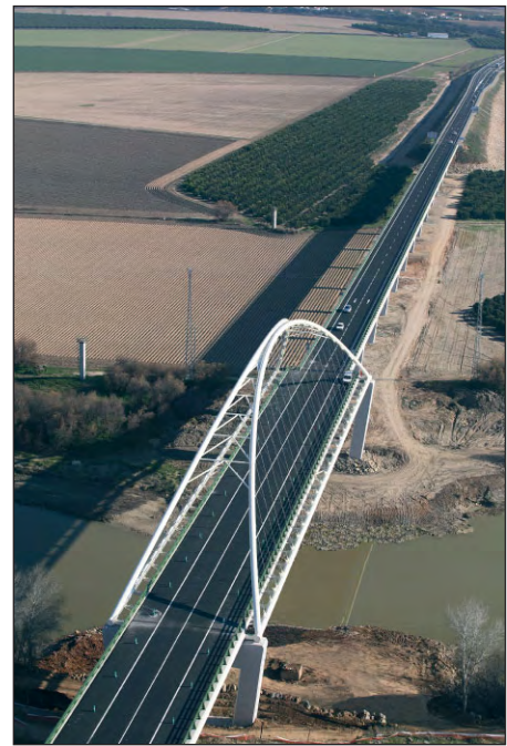
Fig. 6: Aerial view of the bridge
