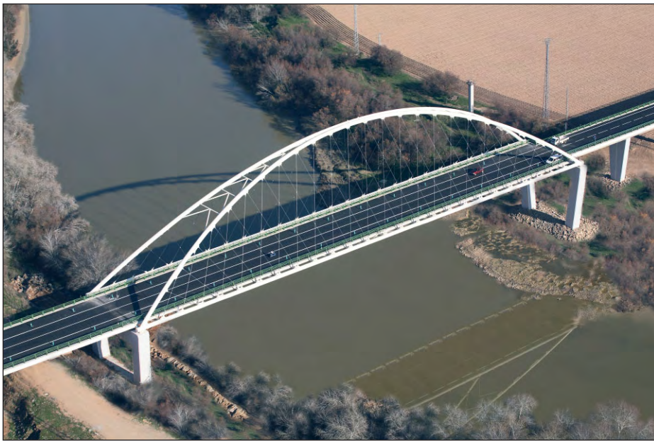
Fig. 4: Aerial view of Palma del Río Bridge over Guadalquivir River
