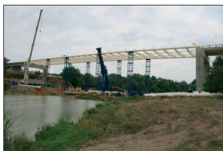
Fig. 13: (a) Erection of the central segment of the deck (b) Concluded view of the deck propped
