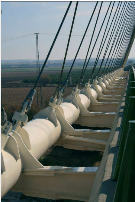
Fig. 9: Anchorages every 5 m
