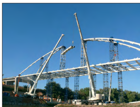
Fig. 14: (a) Erection view of the two inclined arches (b) Close operation
