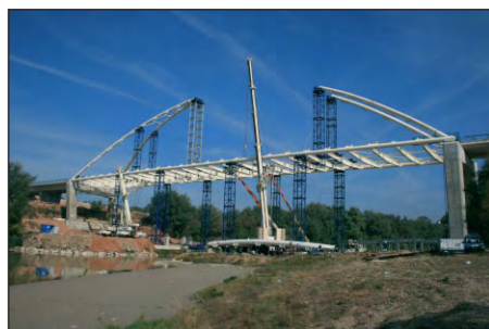
Fig. 14: (a) Erection view of the two inclined arches (b) Close operation
