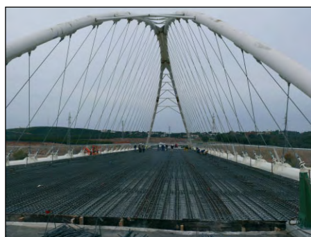
Fig. 15: (a) View of the positioning of the upper precast slabs. (b) The reinforcement of the deck
