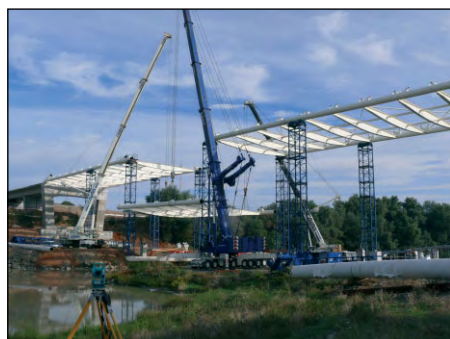
Fig. 12: View of the embankments of both sides of the river and the first segments of the steel framing for the deck
