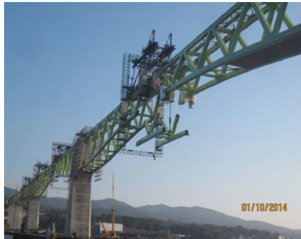
Figure 43. Hoisting the joining segment for span 8.
