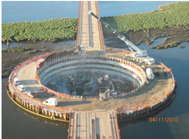
Figure 8. Inner excavation in P5 enclosure.
