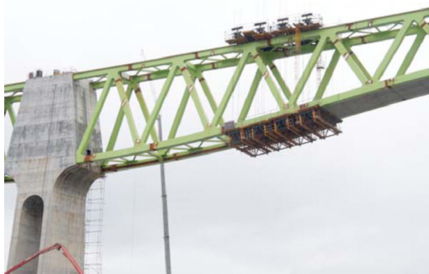
Figure 45. Travelling formwork for casting bottom slab concrete.
