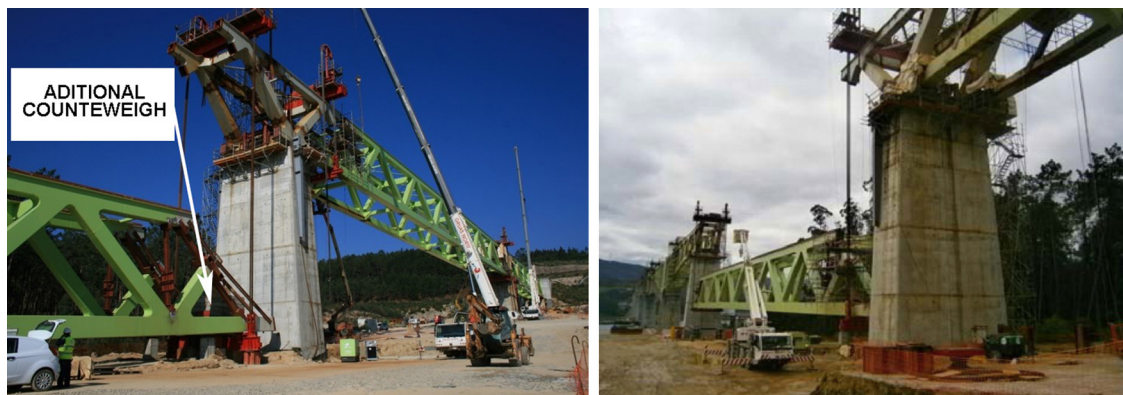
Figure 28. Hoisting sequence for spans 11 (left) and 10 (right).
