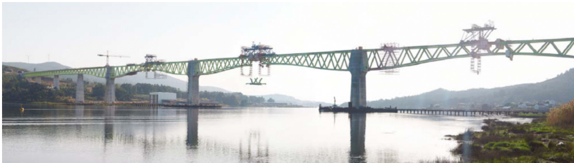
Figure 44. Hoisting the joining segment for span 7.
