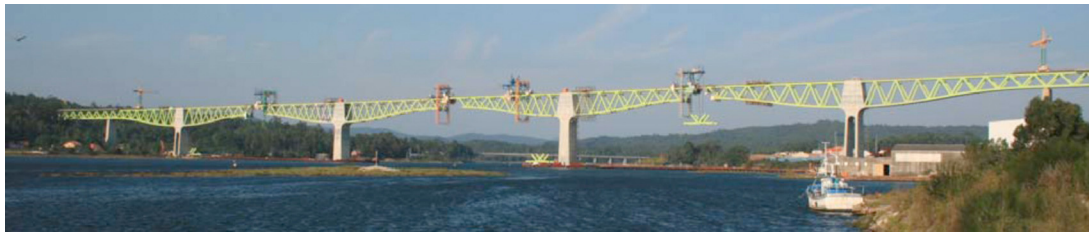
Figure 42. Hoisting the joining segment for span 6.
