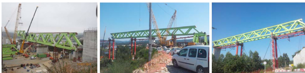
Figure 23. Segment hoisting, first launch and section after launching from P2 to P3.
