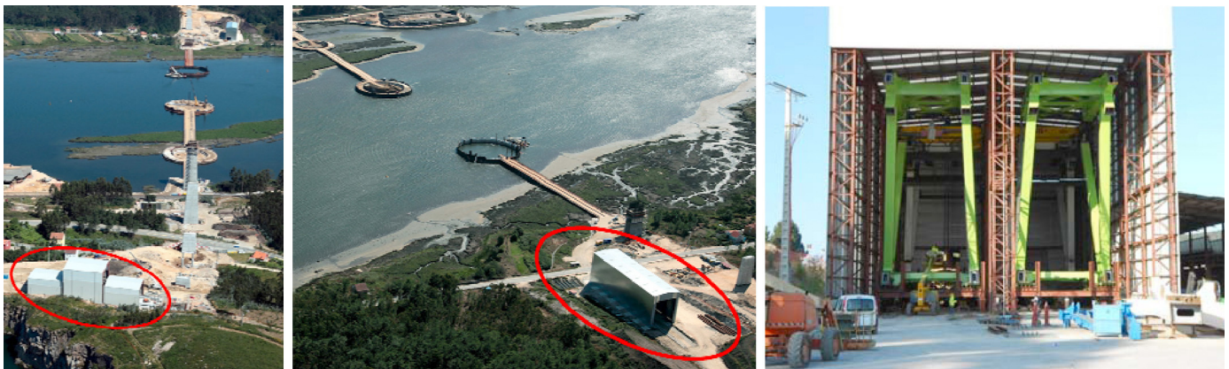
Figure 14. On-site segment assembly bays.
