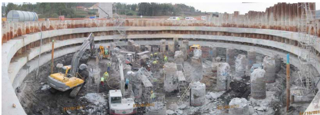
Figure 9. Cutting down P5 foundation pile heads.
