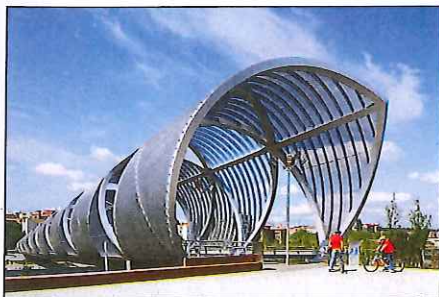
Arganzuela Helix Footbridge, Spain, Pg. 92
