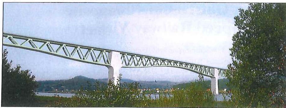
Fig. 2: Lateral view of viaduct over River Ulla
