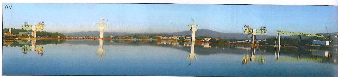
Fig. 12: (a) Approaching spans near abutment 2 (120 + 120 + 80 m) ready for vertical lifting and (b) current state of the works
