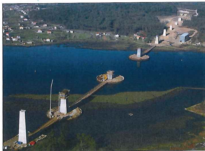
Fig. 7: Aerial view of the construction of the piers inside the river
