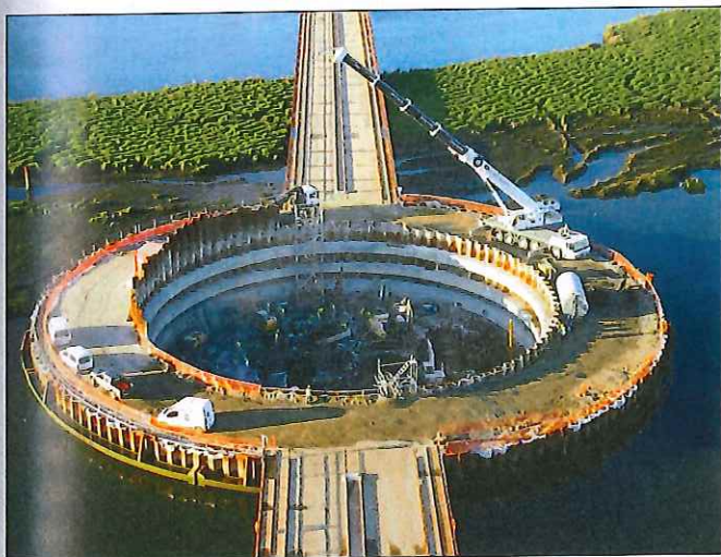
Fig. 6: Execution of the excavation of the pile cap for the foundation of P-5 on the river
