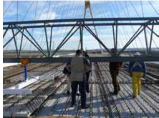
Fig. 23: Positioning of the precast slabs.
