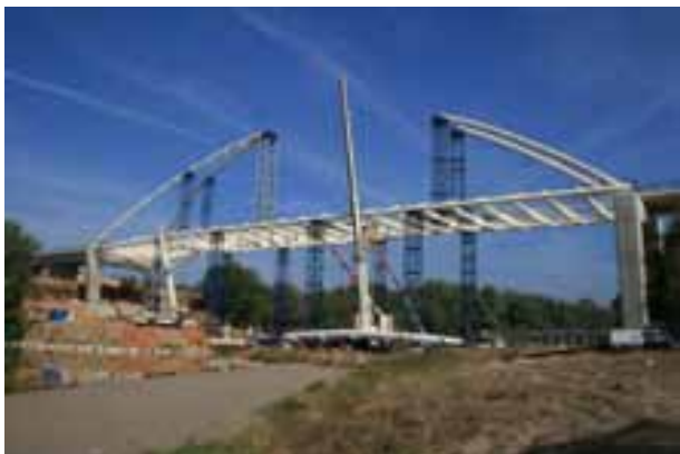
Fig. 20: View during the arches' assembly.
