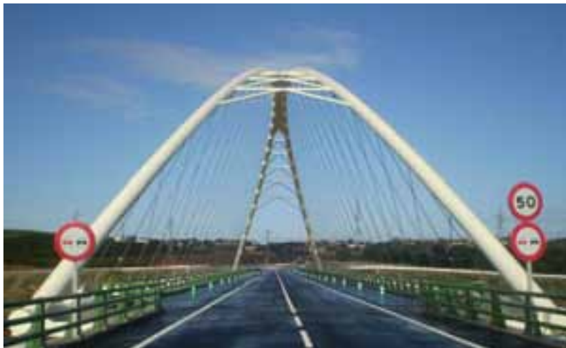
Fig. 16: Frontal view of the inclined arches and the upper bracing.
