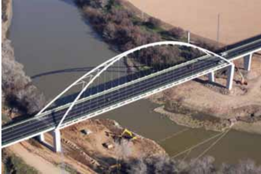
Fig. 13: Aerial View of “Palma del Río” Bridge over Guadalquivir River
