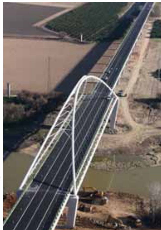
Fig. 15: Aerial view of the bridge
