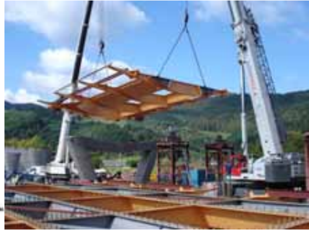
Fig. 11: View of the deck while erection
