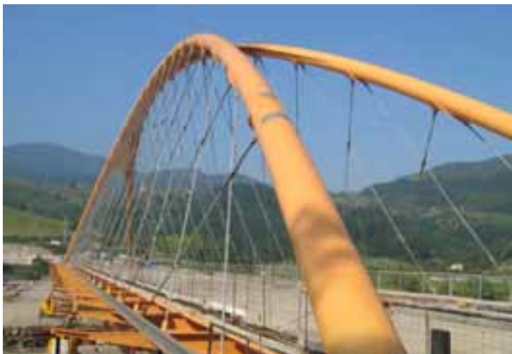
Fig. 24: View of the rod hangers of Deba Bridge.
