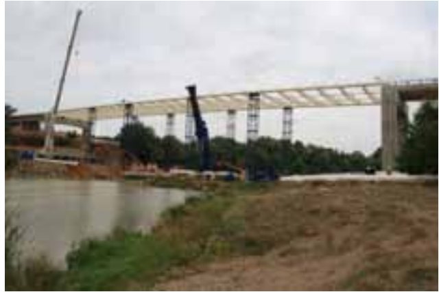
Fig. 19: View of the complete deck supported on provisional piers
