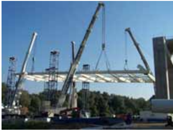
Fig. 18: View of the elevation of one complete segment of the deck
