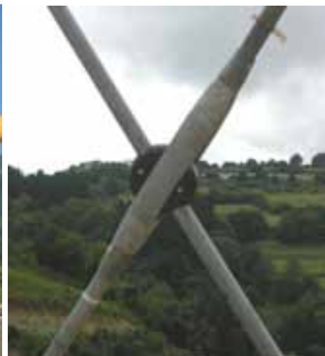
Fig. 25: Detail of the hanger crossing device
