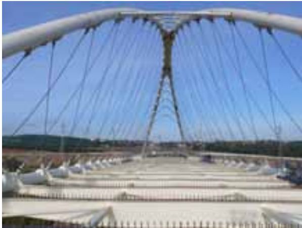
Fig. 22: Fitting of the hangers
