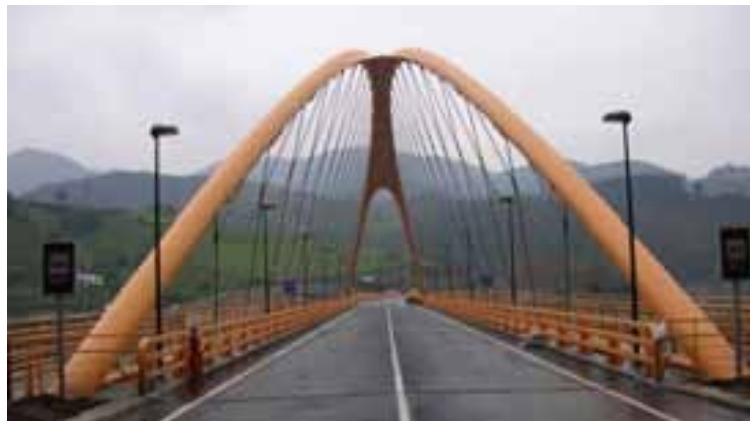
Fig. 9: Front view of the bridge over Deba River
