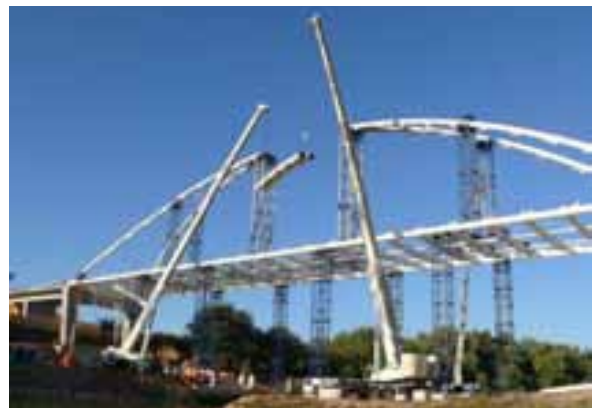
Fig. 21: Arches' crown closing operation
