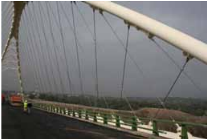
Fig. 26: View of the cable hangers in Palma del Río bridge
