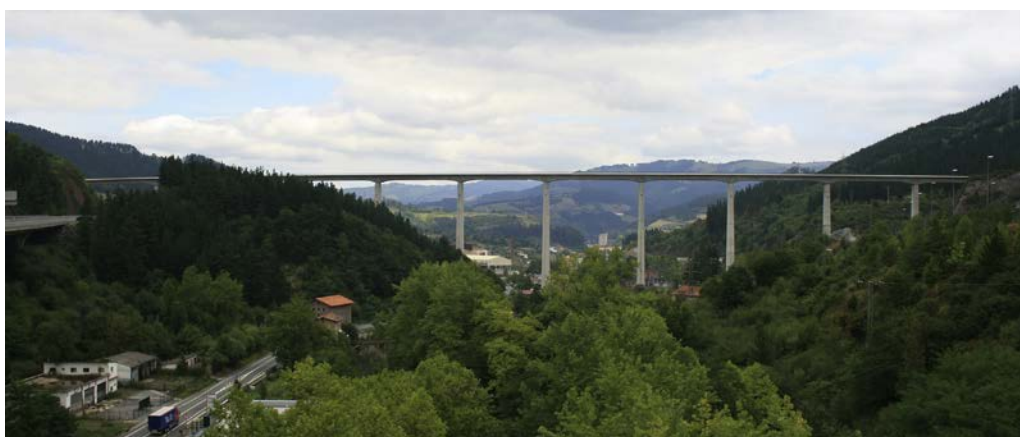
Figure 11. View of finished prestressed concrete viaduct.
