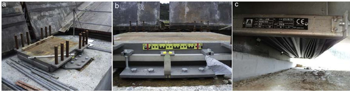
Figure 13. Bearing, ruler-based measuring system and dust cover.
