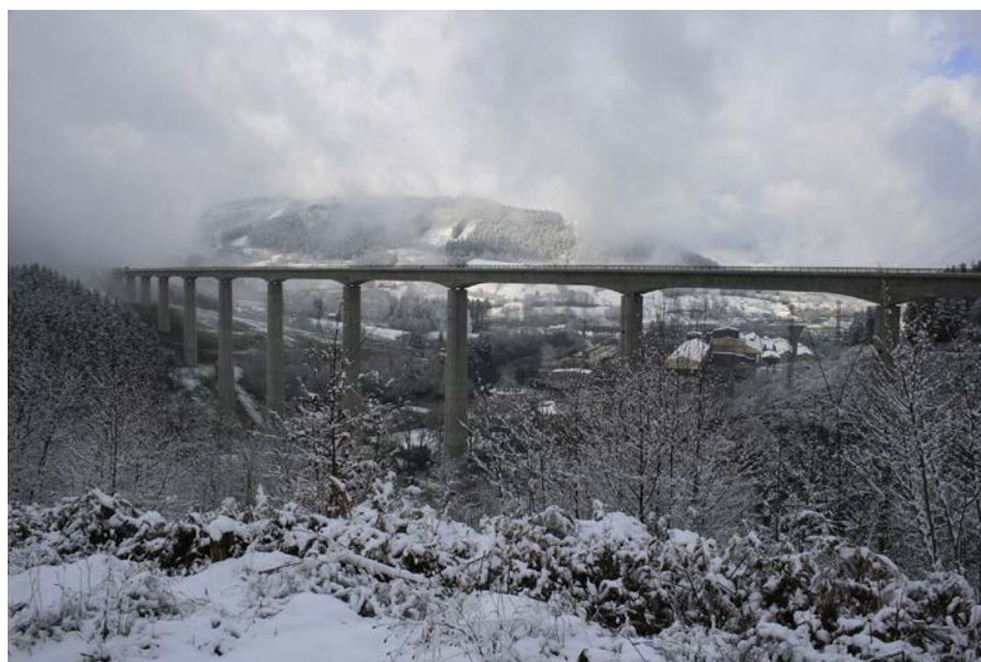
Figure 43. Viaduct during load test with lorries (4 February 2015).
