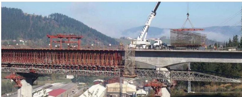
Figure 29. Positioning pre-assembled reinforcement on deck.
